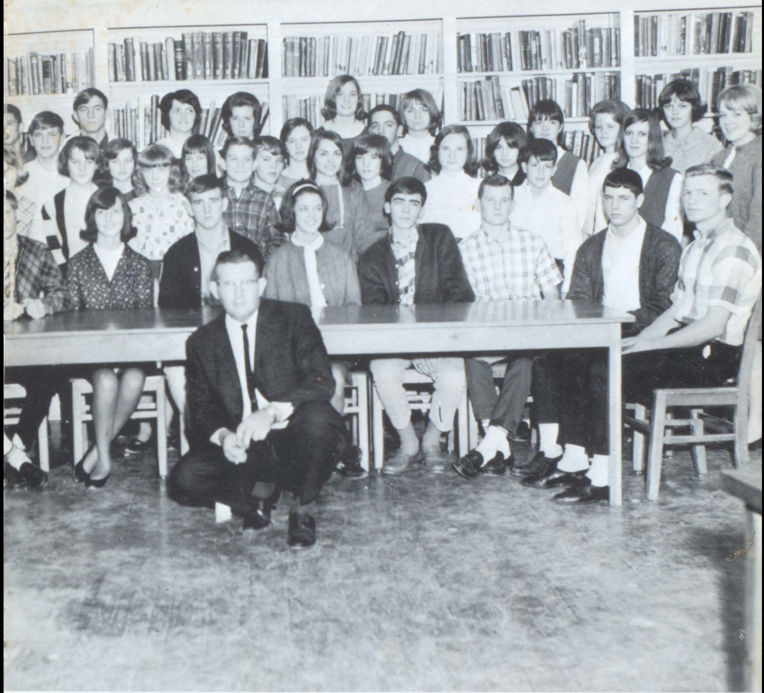
Student Council sells candy each year to raise money for their project. Student Council helped to finance the covered walkway between the Vocational Building and the Elementary Building.
